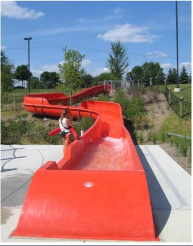
Examples of water slides with a "run out trough".
